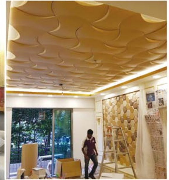
Ceiling in Lobby
