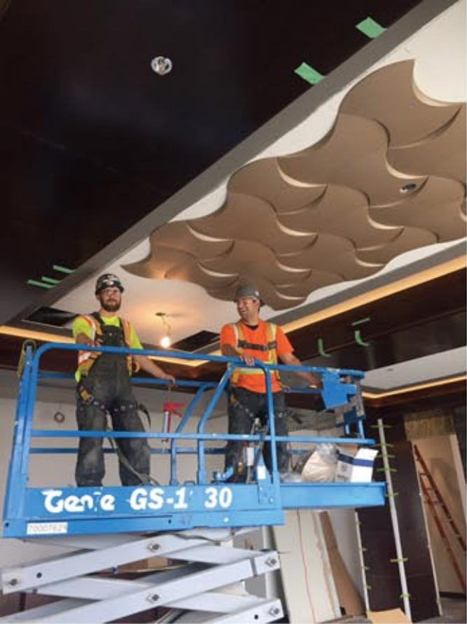
Ceiling in Lobby
